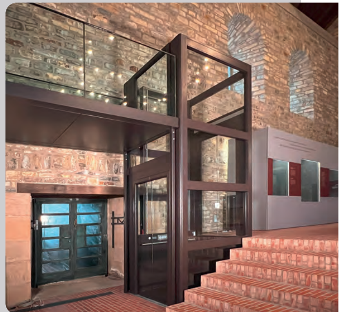
Typical Ganser: Maximum independence thanks to self-supporting shaft
