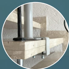
Pillars fixed to the stairs with clamps
