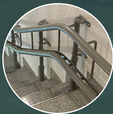
Supports screwed to the wall
