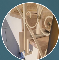
Pillars fixed to the string of the stairs
